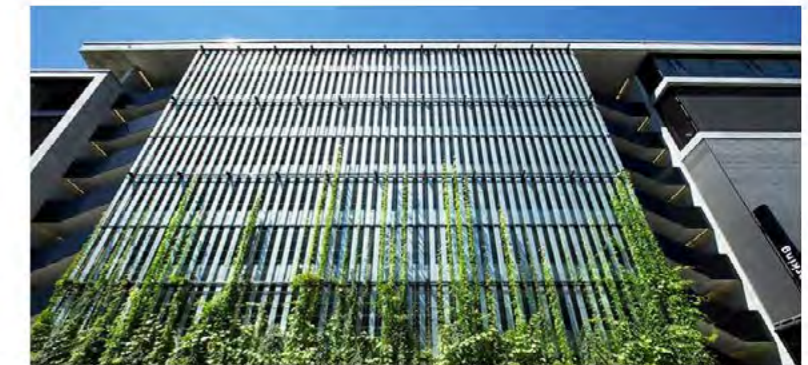
Blank façades to large buildings can have integrated cable systems to grow vines and climbing plants
