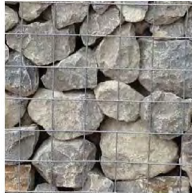
Kentish ragstone gabions can be utilised in marsh areas, potentially to form flood embankment edges or seat walls
