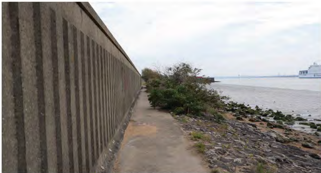
Riverside view at Tilbury Docks, showing sea wall
