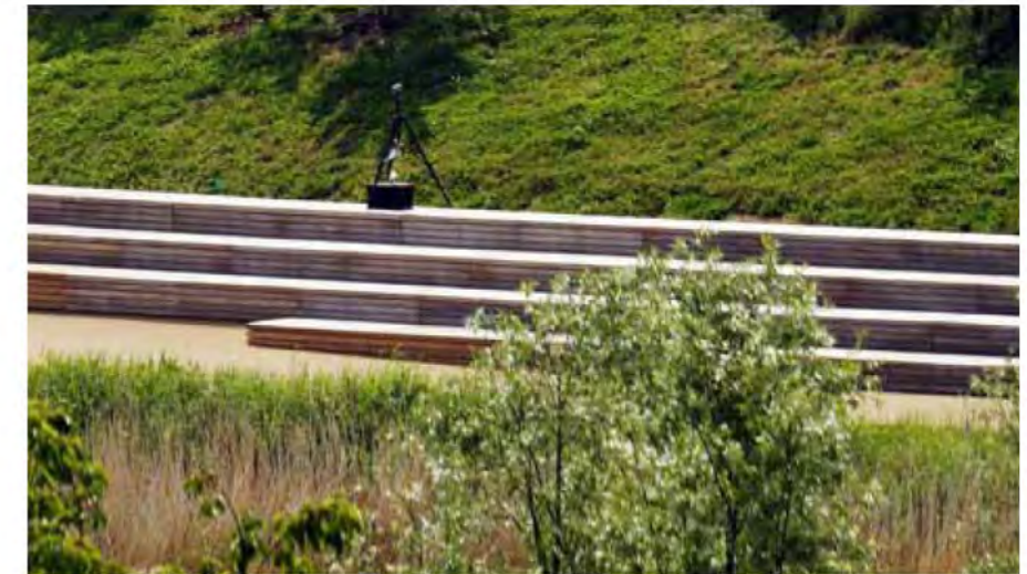
Seating integrated into flood embankment edge
