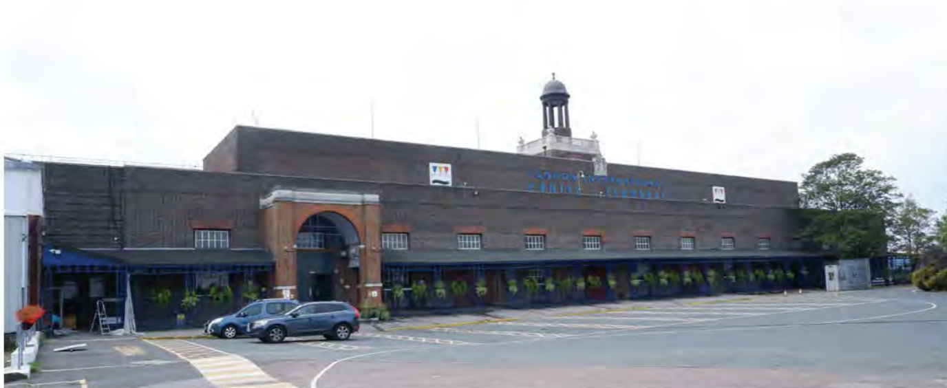
The Grade II* Listed former Tilbury Riverside railway station building at the Essex Site
