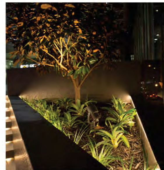
Concealed LED fixtures in planter minimising uplighting
