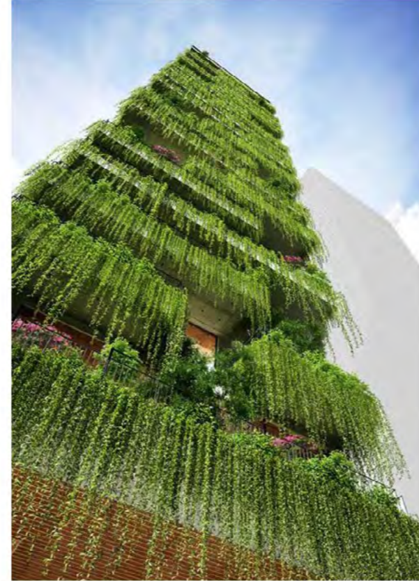
Green building façades
