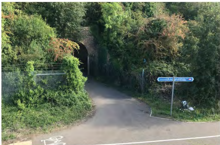
PRoW through embankment tunnel near Ebbsfleet International (DS17)
