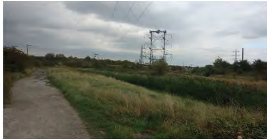
Wider pathway alongside pylons (DS1)
